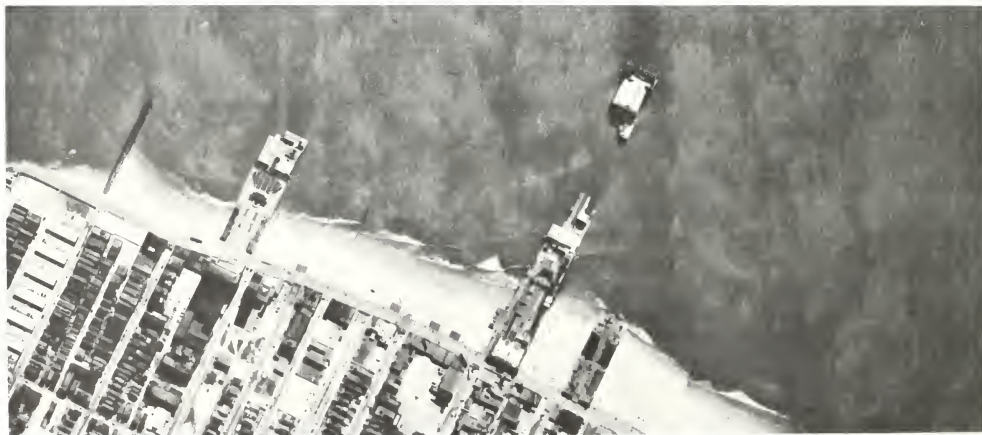
FIGURE 113a.—Aerial photograph taken over Atlantic City, N.J., at 1030 e.s.t. on March 25, 1962, showing damage to Steel Pier by severe tidal flooding of March 6-7. Flight altitude, 10,000 ft; scale 1:20,000.
